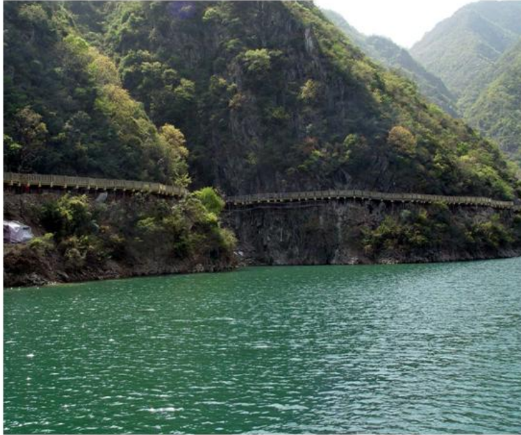
Reconstruction of the Plank Road at the Stone Gate Reservoir
